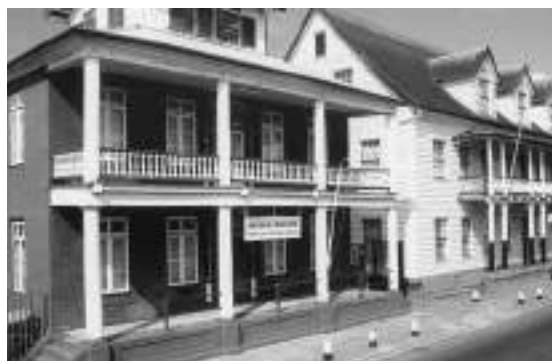
A section of Gravenstraat in the heart of historic Paramaribo (Suriname) that was destroyed by fire some months after this photo was taken in 1996
